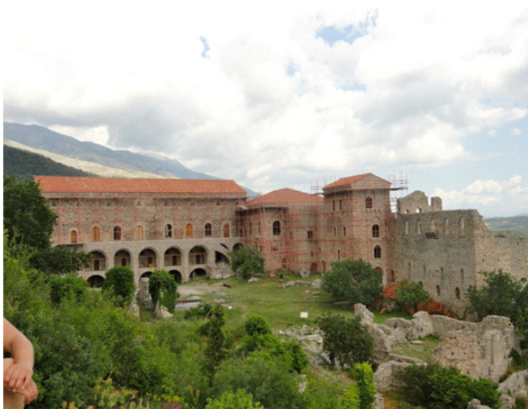
Palace of the Despots under Restoration
