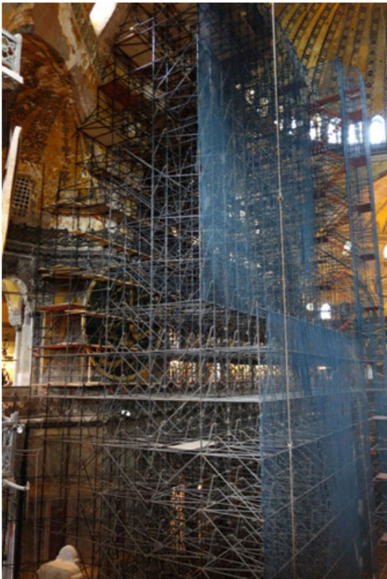
Restoration of the Nave of Hagia Sophia
